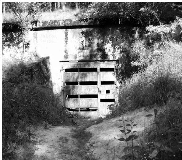
Entrance to one of the Bunkers Now sealed except for access for bats Photo by Robin Ware
